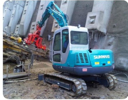
Construction of Foundation Pit in France
