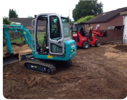
Construction of Family Garden in Europe
