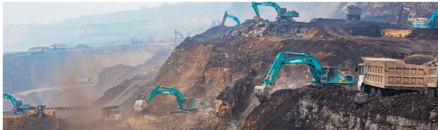
Construction in Open Pit Coal Mine in Shanxi Province
